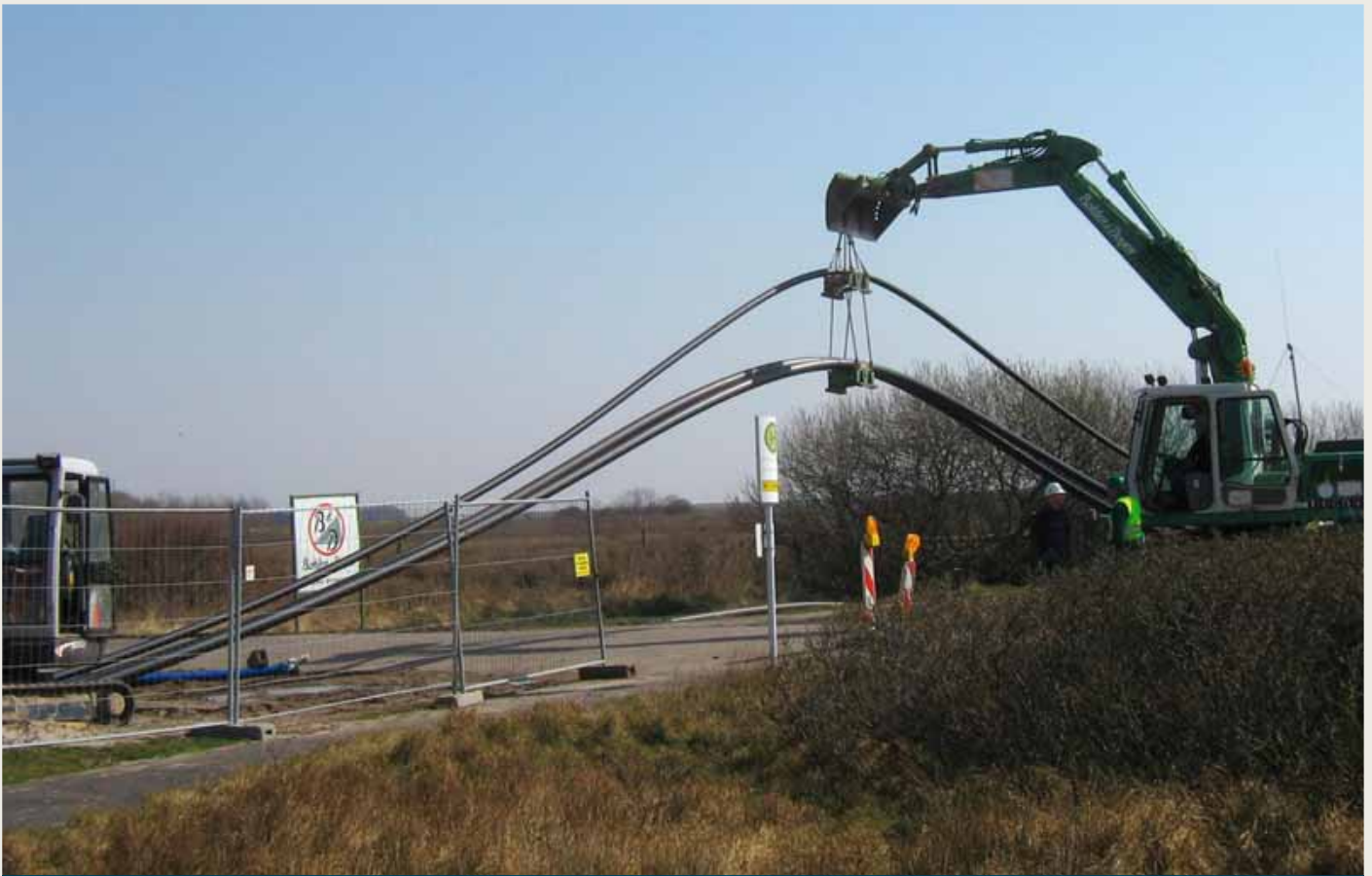
Pulling in the HDPE pipe bundle during the third bore.
